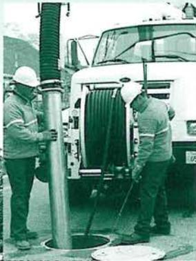
*After the need for maintenance is determined, our crews clean pipes with a giant vacuum and water jet truck, or the pipelines with problems are lined or replaced.*
