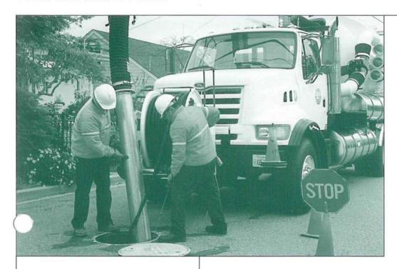
Goleta West crew working with Hydroflush truck that cleans sewer pipelines; photo below shows crew member checking backup power generator. The wastewater collection pipelines are designed to flow primarily by gravity, making them more reliable, with lower operating costs than pumped systems.
