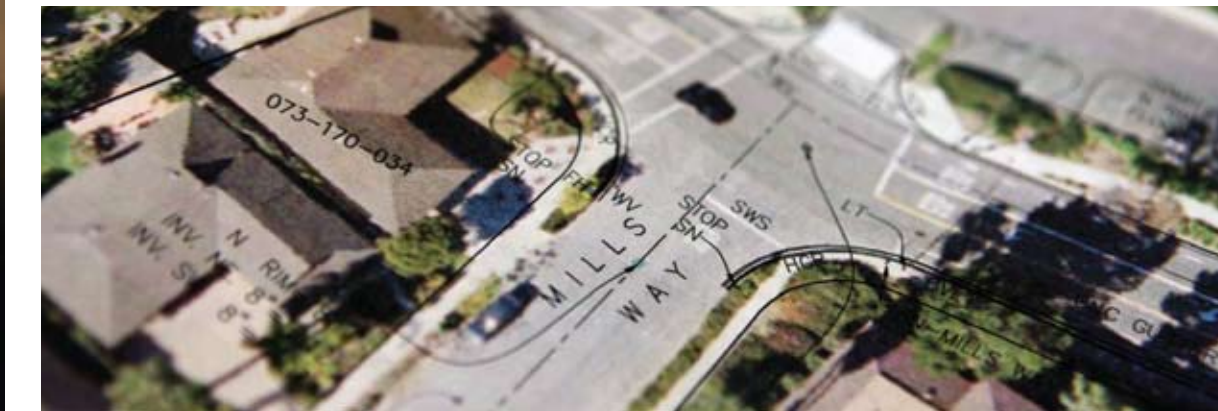
Aerial photo showing pipelines
