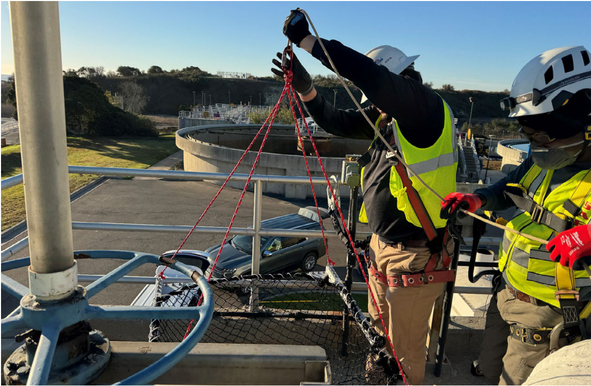
Figure 2.2: SmartBall Extraction Net Being Placed into Position
