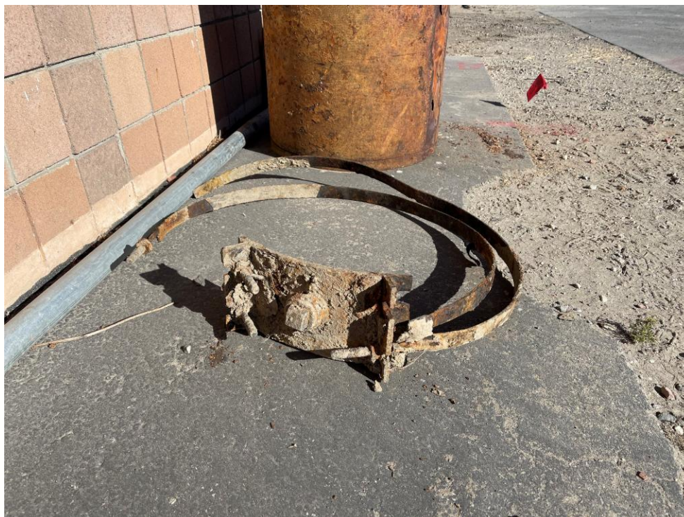
Figure 1-3. Failed ductile iron pipe hot tap adapter removed from the October 2024 spill site
