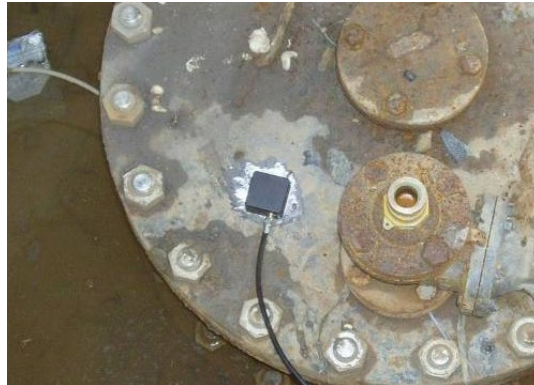
Figure C.7: SMS Adhered to a Flange
