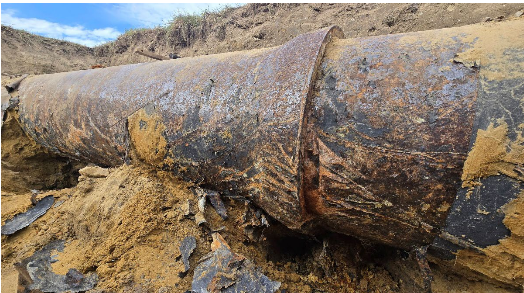
Figure 3. Overview of the 24-inch ductile iron pipe at STA 71+00
