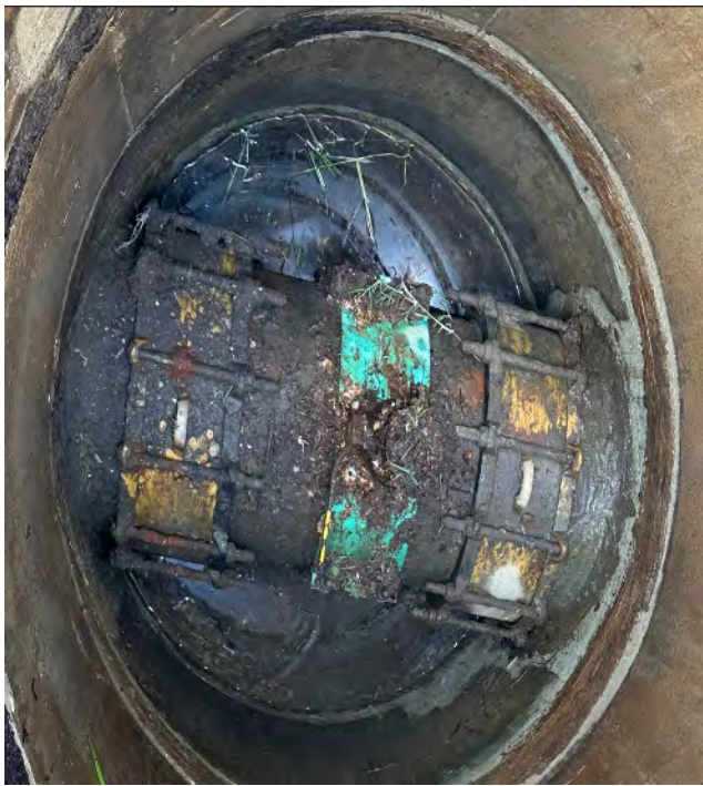
Task B (Photo B13): View inside District 18-inch force main sewer access vault on Santa Barbara Airport; significant corrosion observed on coupling restraining bolts and nuts.
