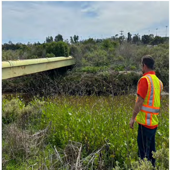
Task C (Photo B8): Inspection of District force main sewer bridge crossing spanning over Tecolotito Creek (view 1); bridge located approximately 700 feet north of District offices.
