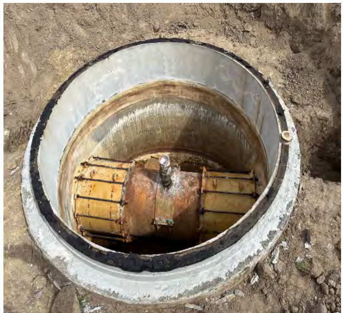
Task B (Photo B18): View inside District 24-inch force main sewer vault located in storage yard; significant corrosion observed on coupling restraining bolts and nuts.
