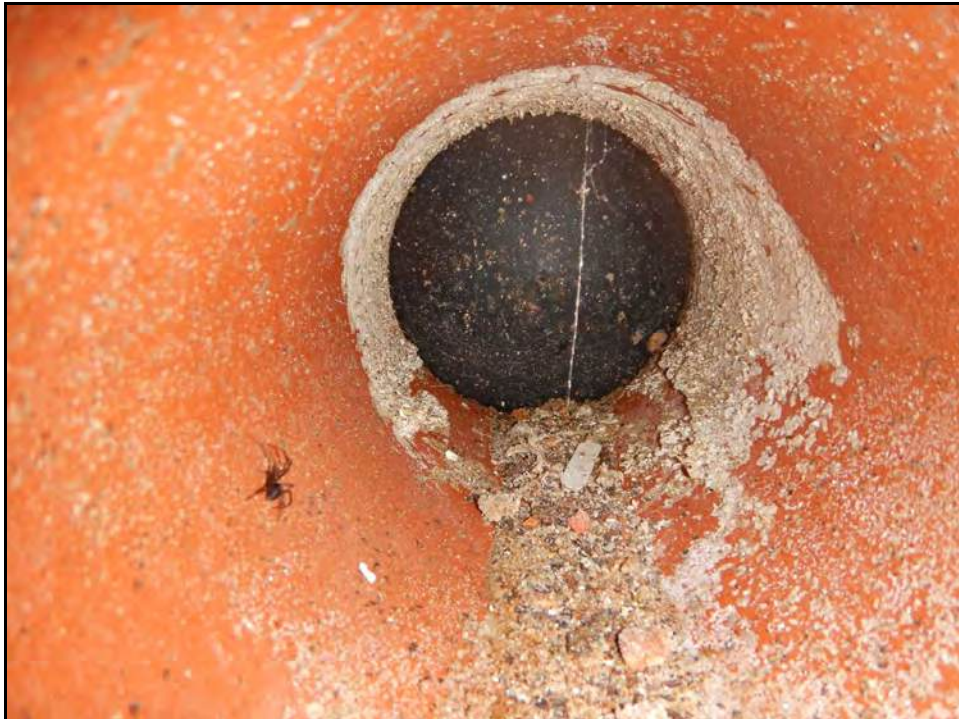
North Lateral Inlet (plugged)
