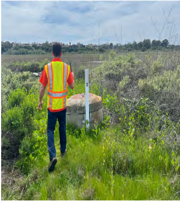
Task B (Photo B5): Inspection of abandoned District force main vault for air release valve (view 1).
