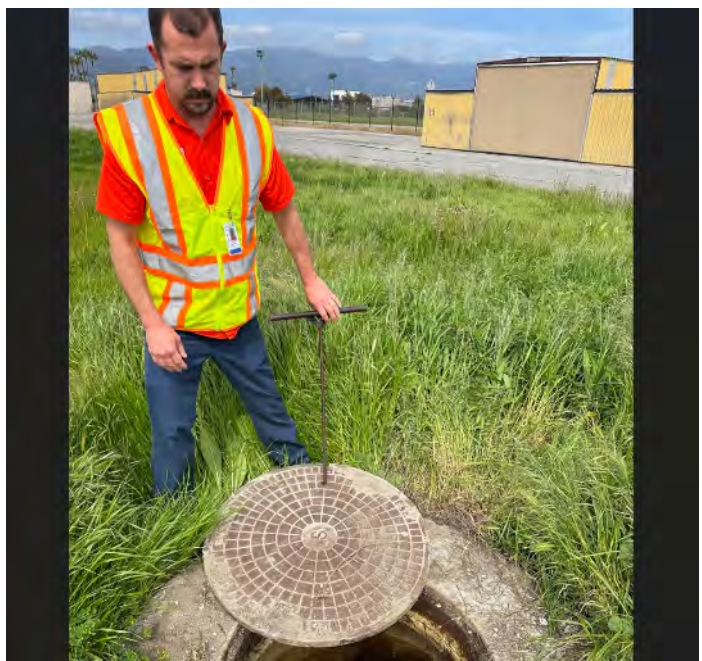
Task B (Photo B12): Inspection of District 18-inch force main sewer vault on Santa Barbara Airport.
