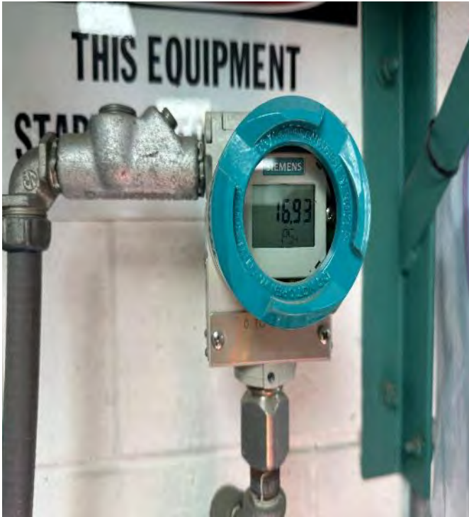
Task F (Photo E5): Inspection of Pump Station 1 force main flow meter.
