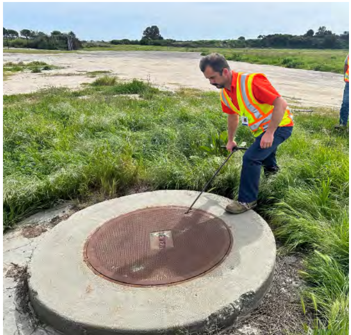
Task A (Photo B10): Inspection of District 24-inch force main sewer vault on Santa Barbara Airport.
