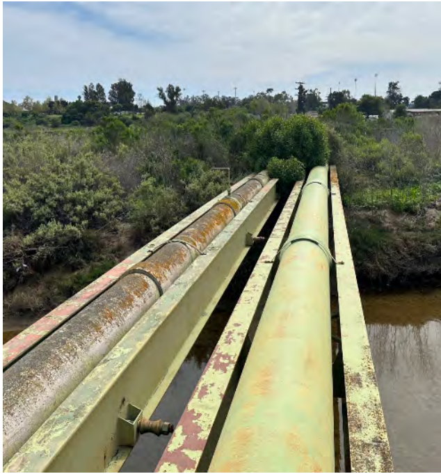
Task A (Photo B9): Inspection of District force main sewer bridge crossing spanning over Tecolotito Creek (view 2); bridge located approximately 700 feet north of District offices.
