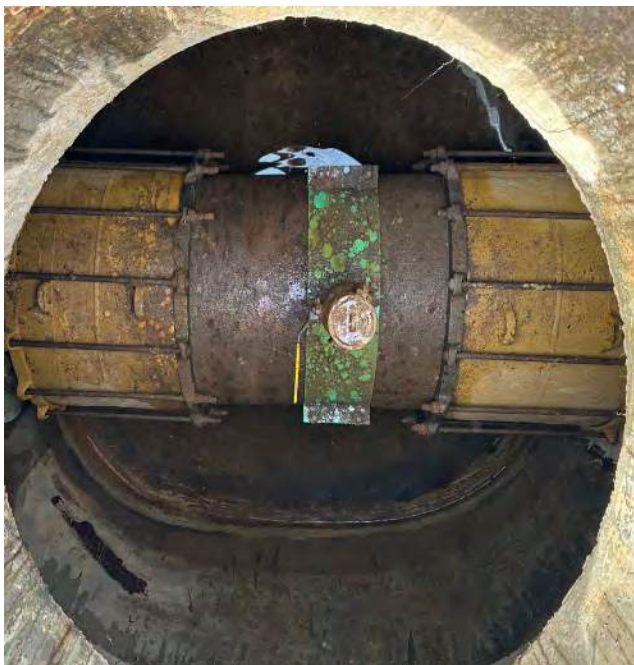
Task C (Photo B11): View inside District 24-inch force main sewer access vault on Santa Barbara Airport; significant corrosion observed on coupling restraining bolts and nuts.
