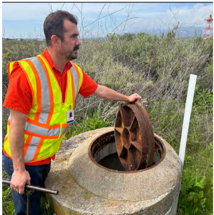
Task B (Photo B6): Inspection of abandoned District force main vault for air release valve (view 2).
