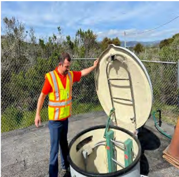
Task D (Photo D3): Inspection of station dry pit access manhole with field staff.
