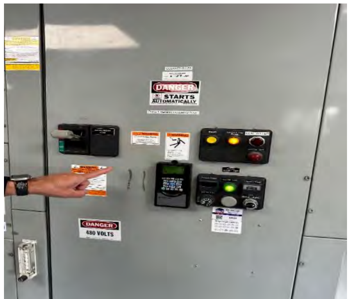
Task E (Photo E4): Inspection of Pump Station 1 Motor Control Center (MCC).
