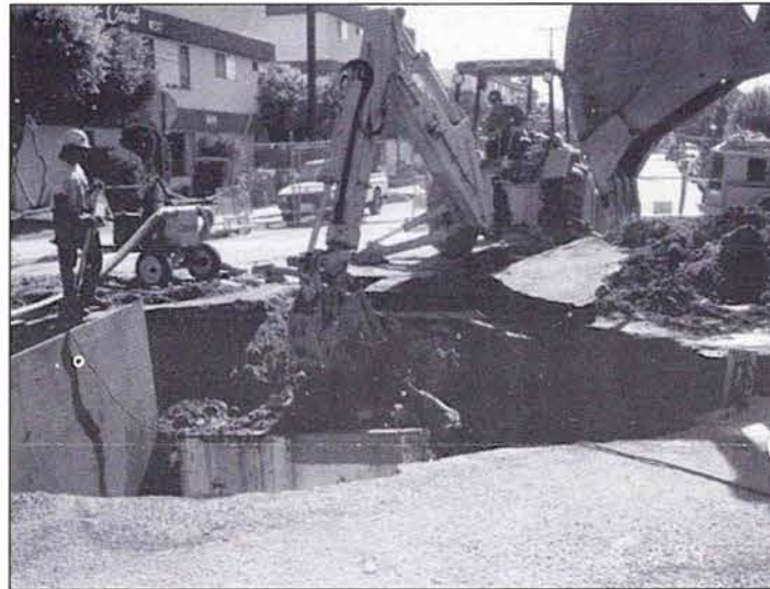
Excavation for manhole construction.
