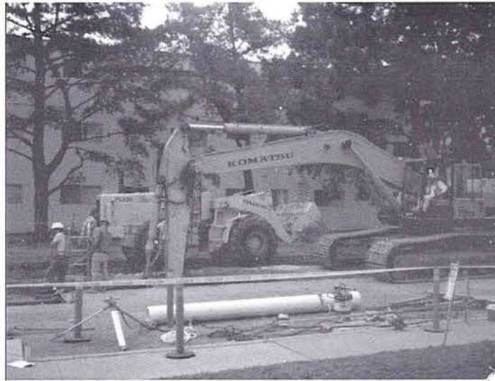
A section of pipe about to be installed.
