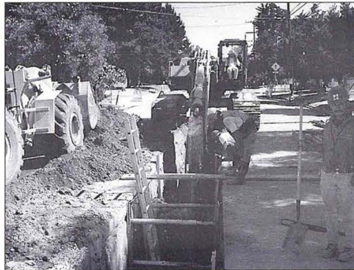
Digging the trench.
