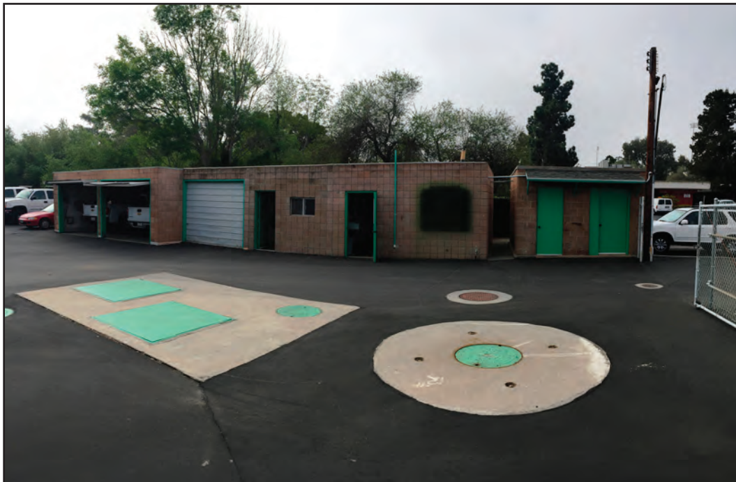
PHOTOGRAPH 2 Buildings to be Removed, Looking South
