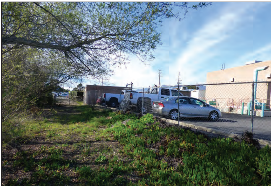
PHOTOGRAPH 4 Project Site South Boundary with Existing Parking and Buildings to be Removed, Looking Northwest
