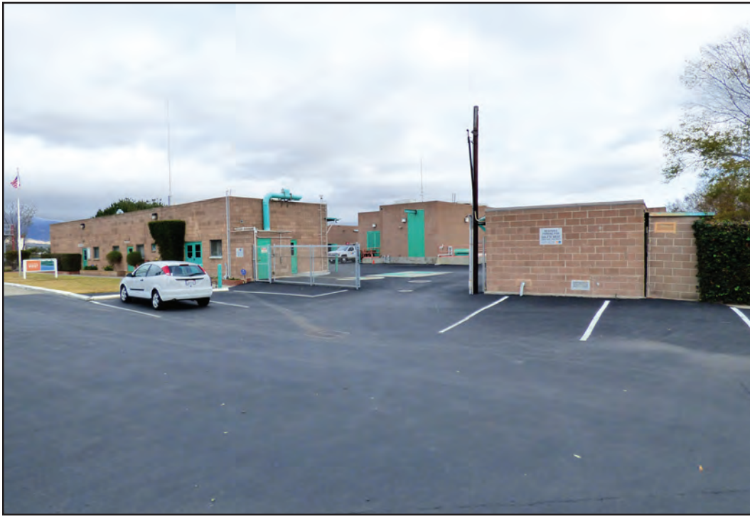
PHOTOGRAPH 1 Existing Buildings with Existing Administration Building on Left and Buildings to be Removed on Right, Looking Northeast
